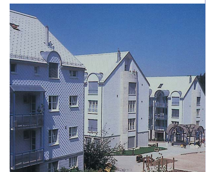
A building in which vynlon is used as a cement reinforcing agent
