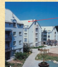
Roof slate made with vynlon-reinforced cement
