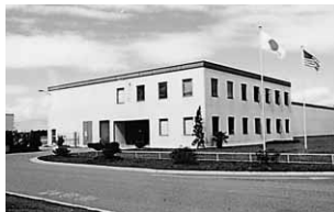
Factory for nonwoven fabrics of Kuraray Chicopee Co., Ltd. (now Kuraflex Co., Ltd.)
