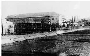
New laboratory of Okayama Plant
