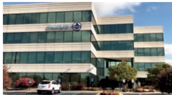
MonoSol Headquarters in Indiana, U.S.A.
