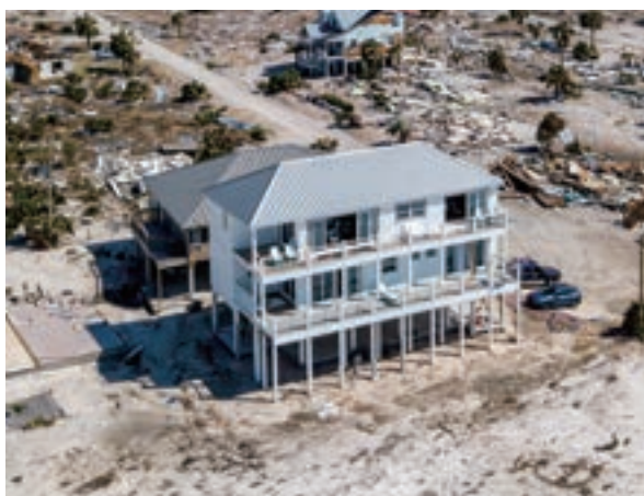
Houses that survived hurricane destruction (Mexico Beach) using Trosifol® for windows and SentryGlas® for doors
