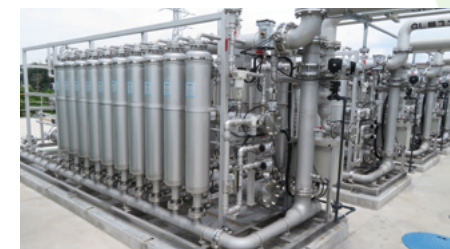
GL module units installed at Kurashiki Plant
