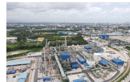
Aerial view of the new plant
